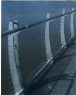
Railing light - Type I railing, illuminated
